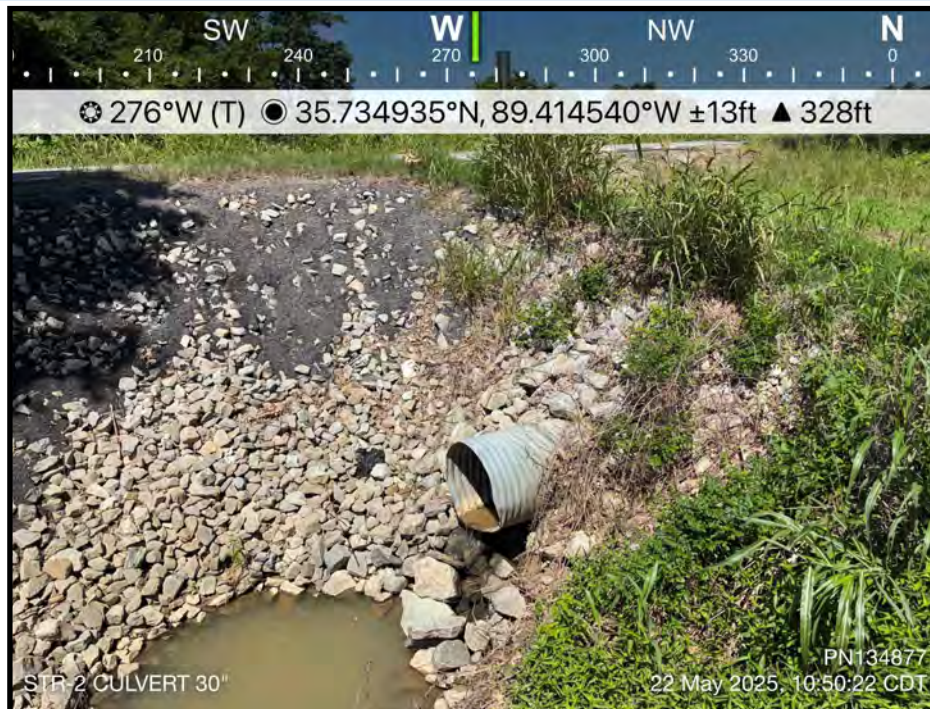
Photo 47: STR-2 culvert 30", under farm field access, 145' north of STR-1 (Otter Creek)
