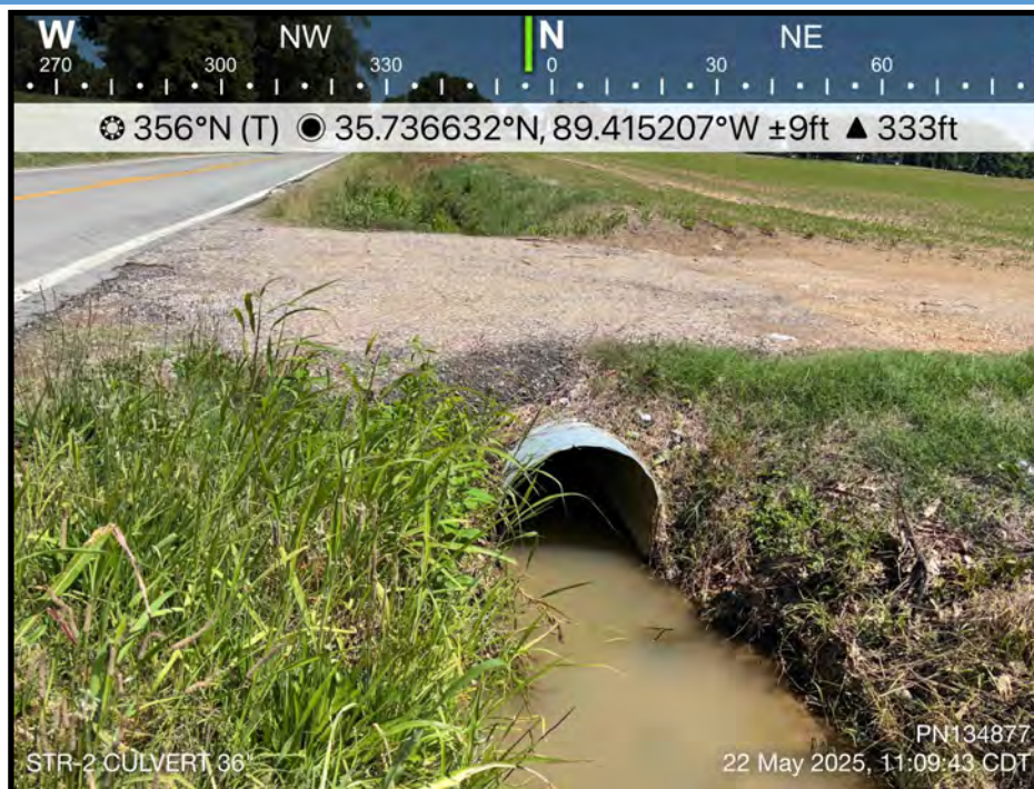
Photo 48: STR-2 culvert 36", under farm field access, 940' north of STR-1 (Otter Creek)
