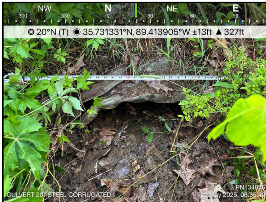
Photo 9: WWC-1/UDF-1 Culvert under farm field access
