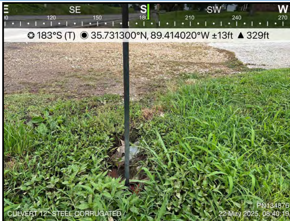
Photo 6: Culvert 12" steel corrugated under driveway to house 2507 Forked Deer Road
