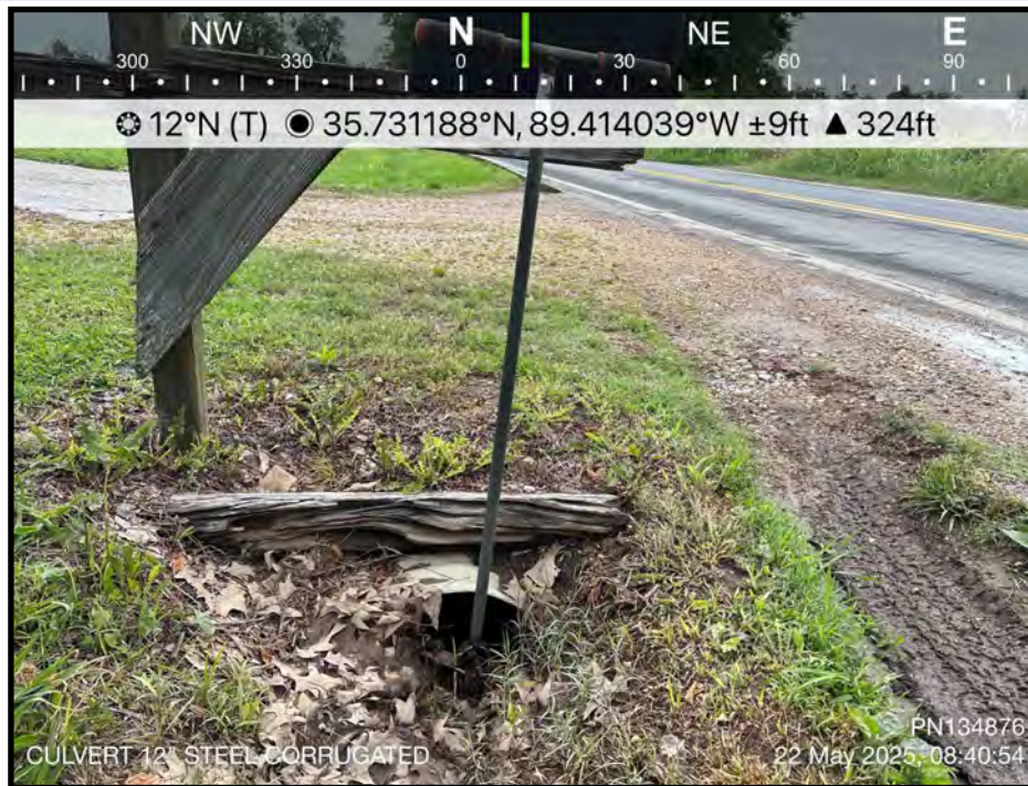
Photo 5: Culvert 12" steel corrugated under driveway to house 2507 Forked Deer Road
